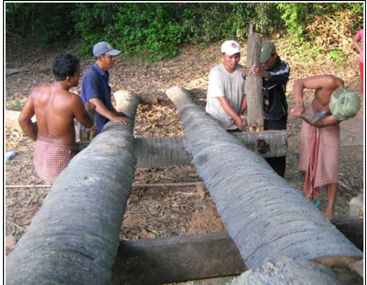
Church members build a bridge for their community.
